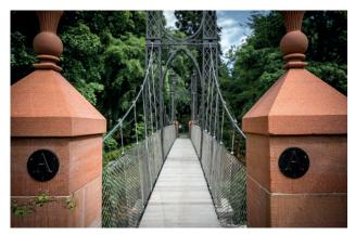
To realise Tom Stuart-Smith's vision for the new access to the castle, Kishorn Heritage constructed a series of roads, a suspension bridge with stone parapets and various connecting terraces, courtyards and paths. All stone used on this project was quarried locally and hand-dressed on site where at all possible. The large courtyards were finished using reclaimed original granite setts from the streets of historic Edinburgh.
